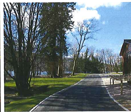
Fallbarrow Park, Windermere: Completed CellWeb TRP® Installation
