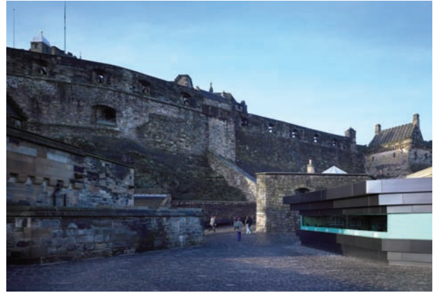
Reception Centre, Edinburgh Castle, Gareth Hoskins Architects, 2007
