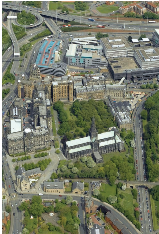
Aerial view of the Cathedral precinct with the Royal Infirmary complex to the north
