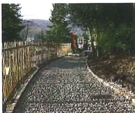
Fallbarrow Park, Windermere: Prior to CellWeb TRP® Installation
