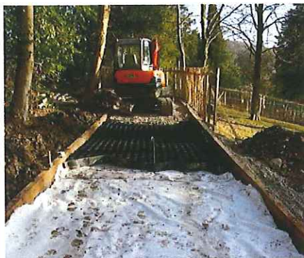
Fallbarrow Park, Windermere: CellWeb TRP® Installation
